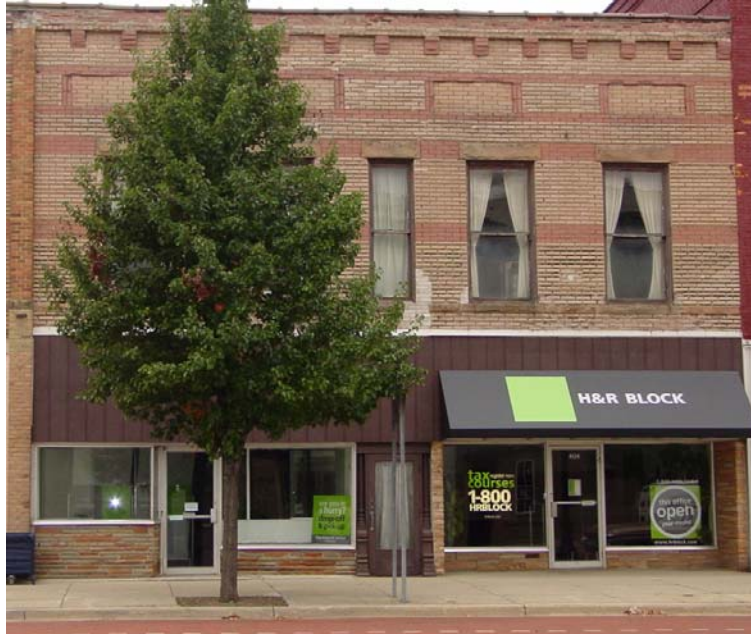
FIGURE 9. H & R Block is an example of a service business that should utilize vertical space
